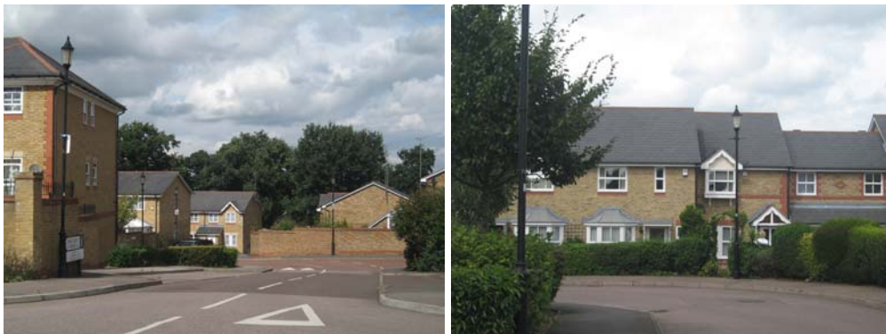
Housing development in the Conservation Area, in the area proposed for de-designation
